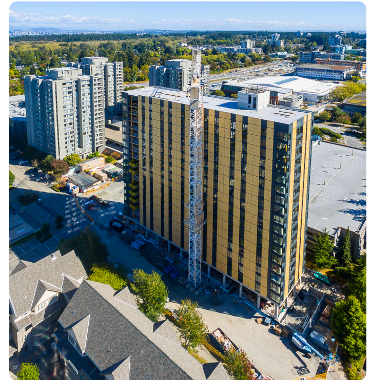
Brock Commons Tallwood House Credit: naturallywood.com Photographer: KK Law ( flickr.com )
