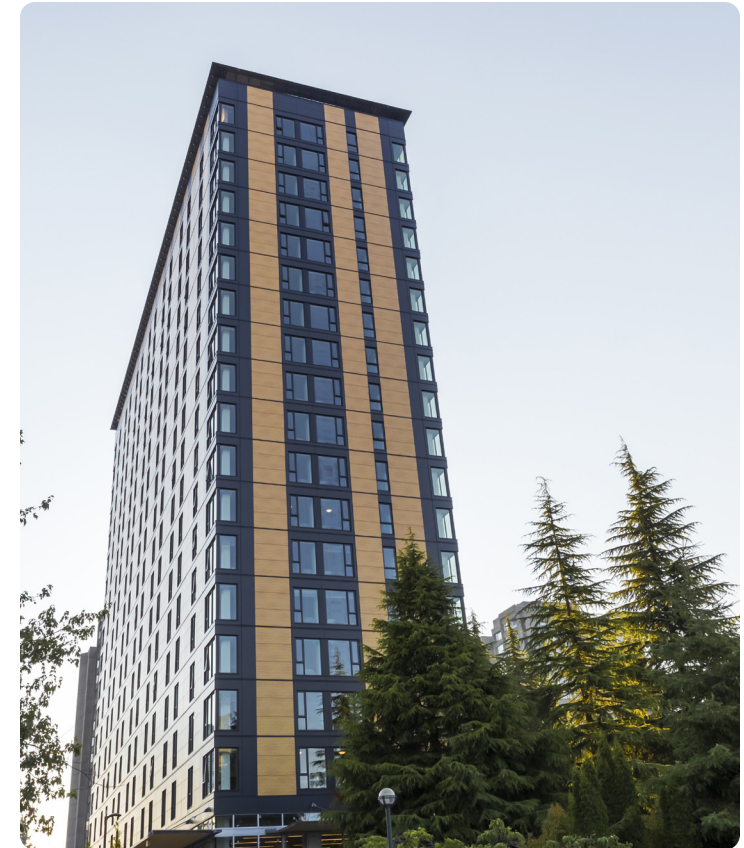
Brock Commons Tallwood House - Photos courtesy of naturallywood.com Photographer: Brudder ( flickr.com )
