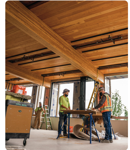
PAE Living Building - ZGF Architects Photographer: Dan Bihn
