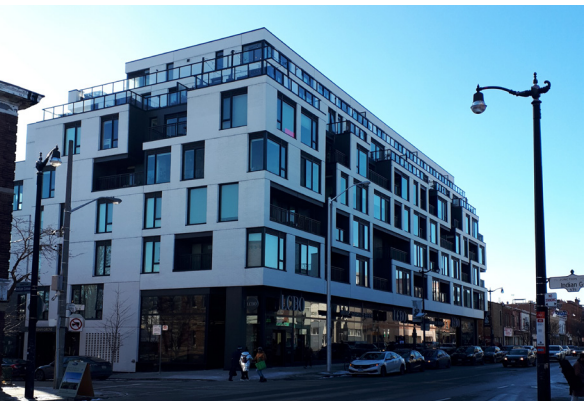
Image: Duke Condos (BDPQuadrangle Architects) Thomas Noussis, Photographer Duke Condos is a 7-Storey, concrete-framed residential building with retail along avenue at grade. The structure allows for distinct, horizontal massing transitions with a variety of terraces, step-backs, and over-hangs breaking up the form and adhering to neighbourhood zoning and planning requirements.
