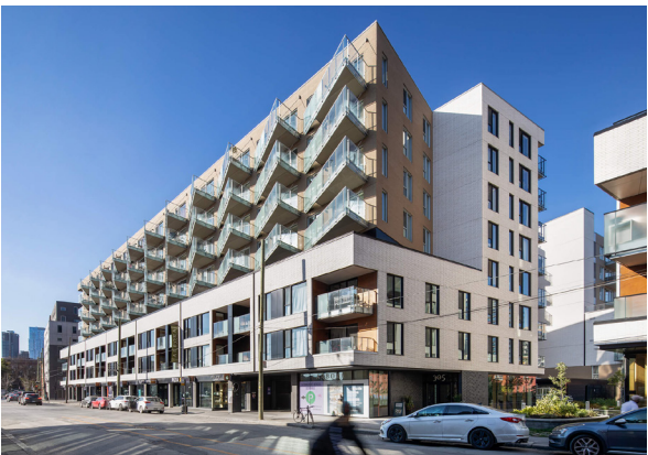
Image: Arbora Apartments (LeMay, CHA, Provencher-Roi Architects) Adrien Williams, Photographer Arbora Apartments combines a 3-storey concrete podium with 5 storeys of CLT/Glulam Framed apartments above. Note the distinct, sheltered transition between pedestrian level uses provided by concrete frame below, and the regularity of the timber-framed floor plate of the apartments above.
