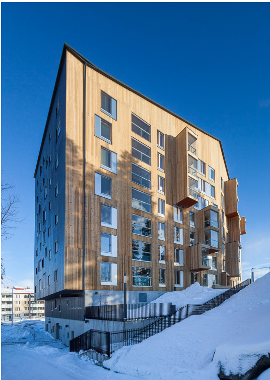
Image: Pukkoka Housing Block (OOPEAA) Mikko Auerniitty, Photographer Pukkoka Housing complex is a trio of gabled bar buildings responding to an irregular site. The design inflects rectangular CLT 'wings' at a central atrium, resulting in a dynamic form with a plan much like a conventional bar.
